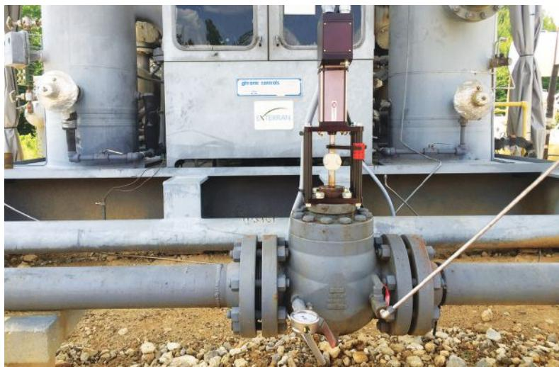
In addition to the controller bleed rates, leaks and malfunctions must be considered as a potential gas-venting source. Leaks from the various tube joints or other points within the tubing network are possible due to worn gaskets or loose fittings. Malfunctions within the controller are possible because of foreign material blocking the nozzle, creating a continuous bleed or excess moisture in the supply gas, which can cause nozzle corrosion.
